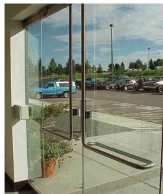
Retrofit installation of Smart Touch replacing mechanical panic
